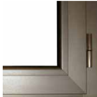
Cerniera a vista Visible hinge
